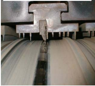
250 MW End Packing – After 17 months
