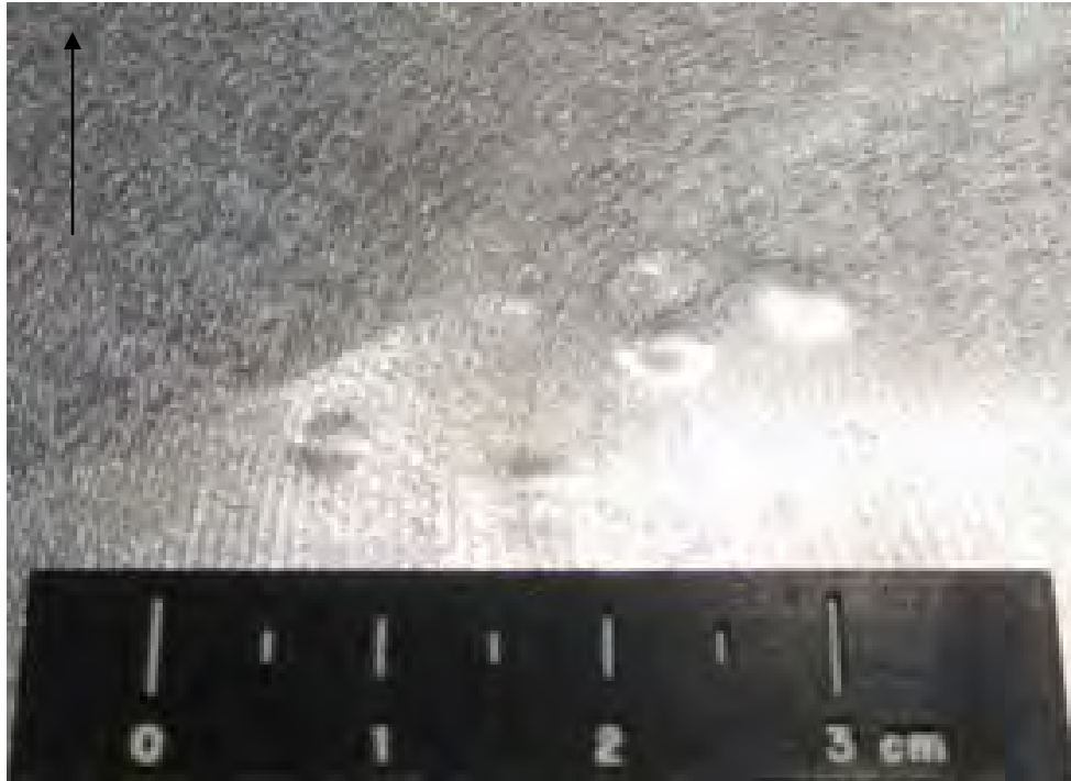
Figure 406 Close-up Oblique Side View of Damage on Back Side of Rear Wall (scale in 5mm increments / black arrow indicates flight path of projectile)
