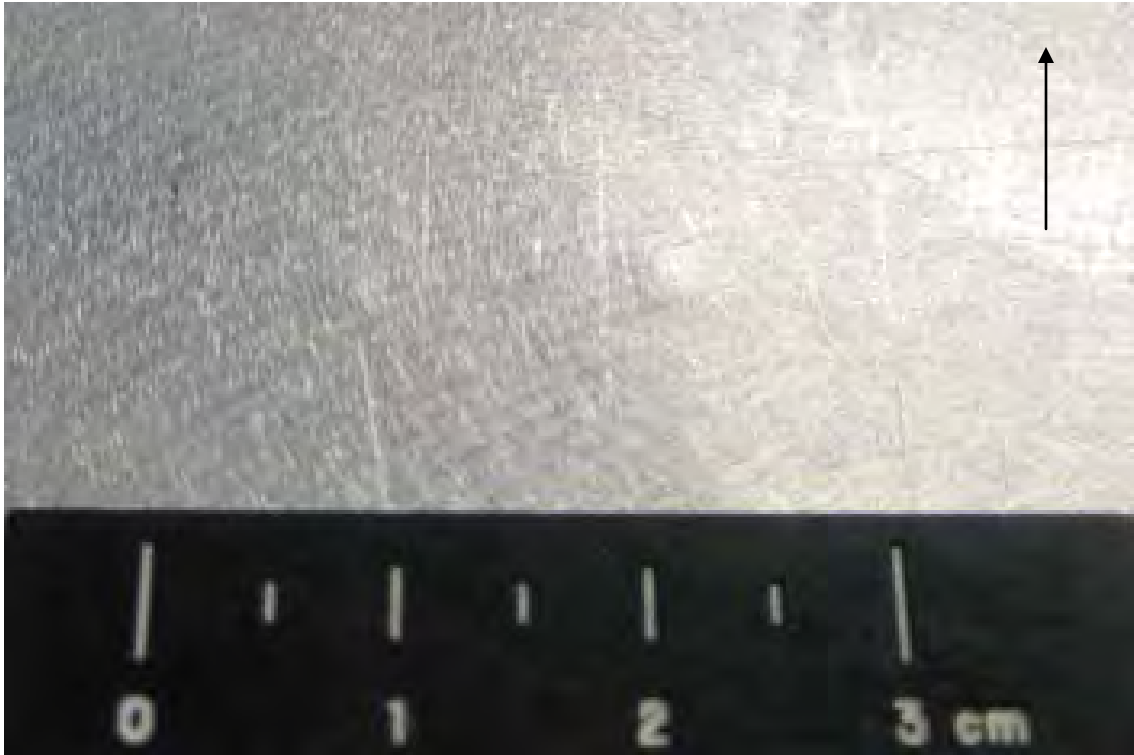
Figure 485 Close-up Oblique Side View of Damage to Back Side of Rear Wall (scale in 5mm increments / black arrow indicates flight path of projectile)
