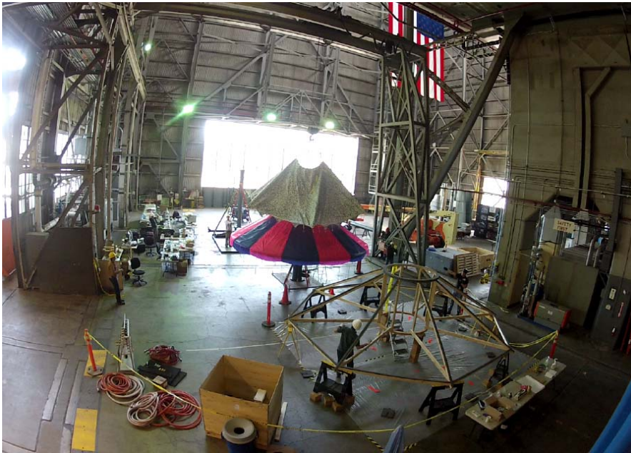
Aerocover Transferred from Integration Fixture to 6 m HIAD using overhead crane in NFAC high bay
