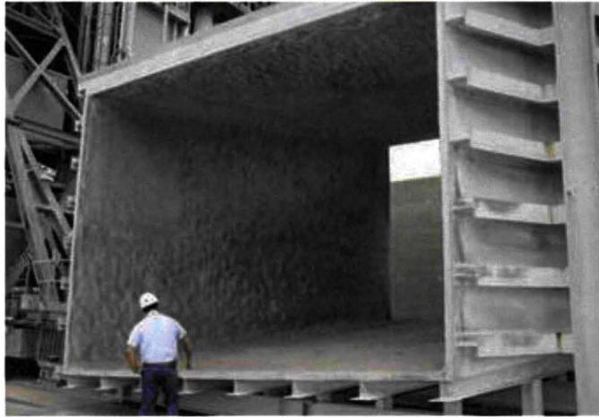
**Figure 33. Side Flame Duct at LC 17B**
