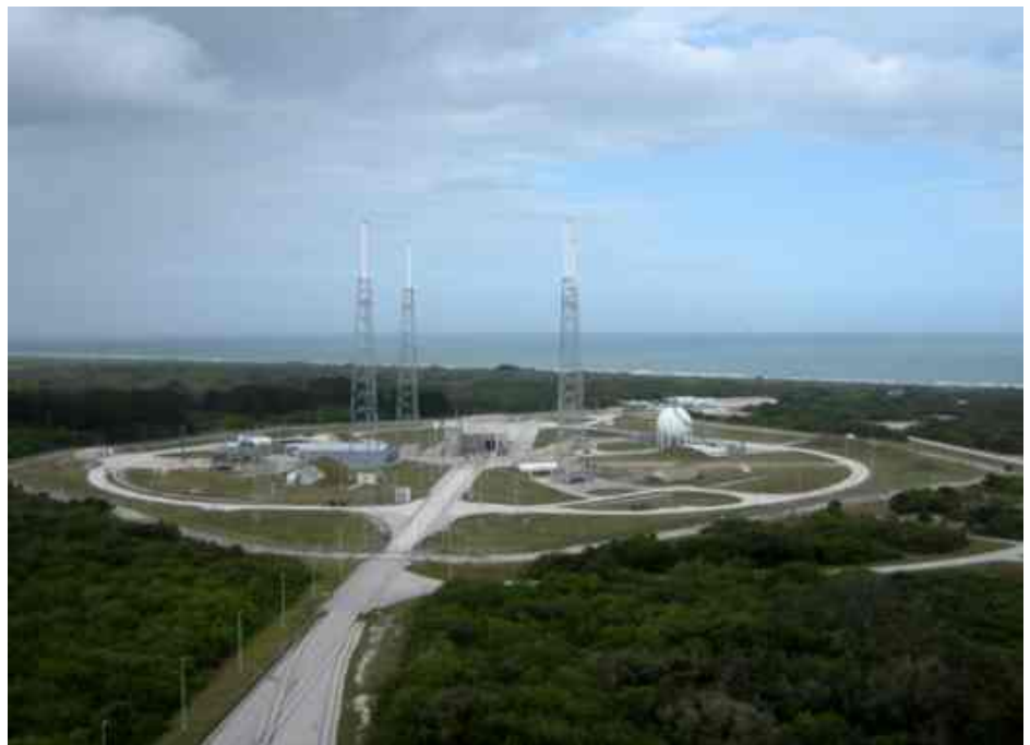
Figure 14-2: Space Launch Complex 41 (SLC41) at Cape Canaveral in Florida, Launch site of LRO/LCROSS. 3
