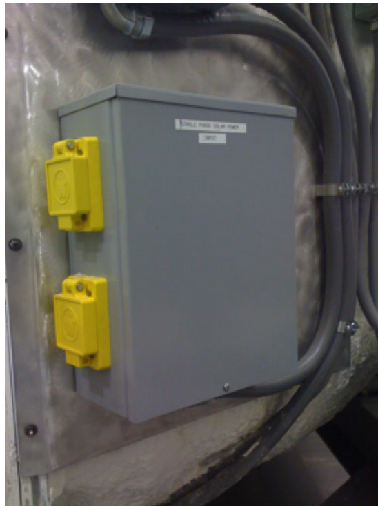
Figure 19.—Photovoltaic (PV) power systems junction box and plugs.
