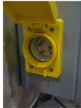
Outdoor-rated twist lock L5-30 plugs
