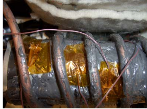
Figure 10. Compressor cooling coils.
