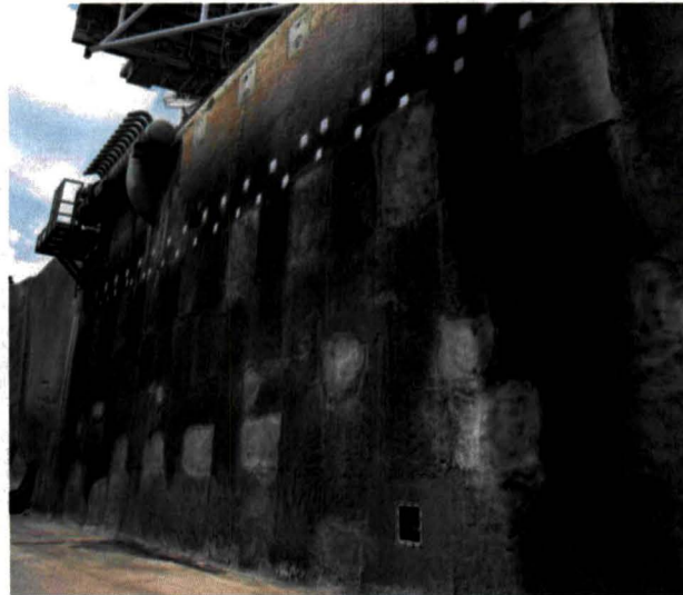
Figure 1. Flame trench wall repairs at Pad 39A
