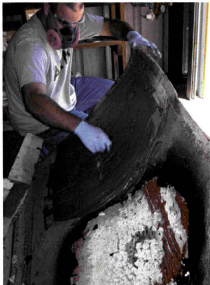
James Captain removing AMTS paste from surface
