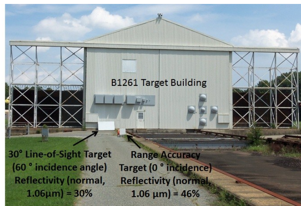
Figure 8. LaRC LDTR 30° LOS target board used for testing at the non-zero incidence angle planned for the maximum range point of the approach trajectory.
