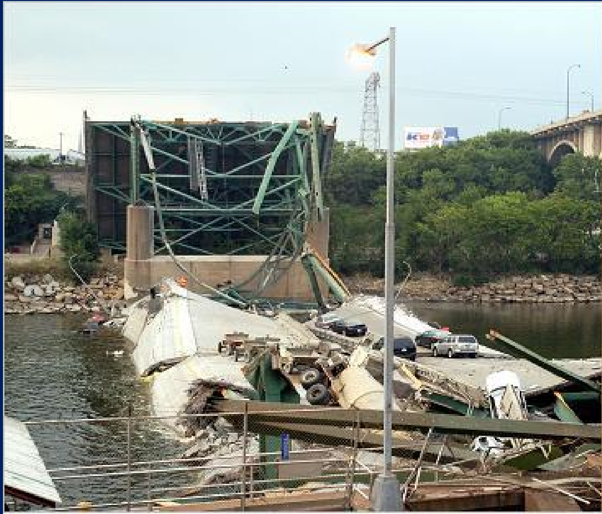
Official Minnesota Department of Transportation investigation photo of the I-35W bridge collapse in Minneapolis, taken Aug. 3, 2007.
