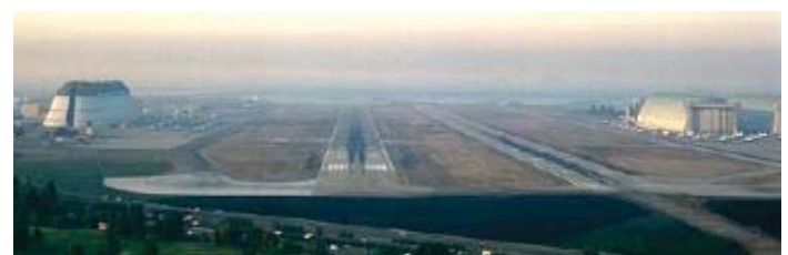
Moffett Federal Airfield with Hangar 1 on the left.
