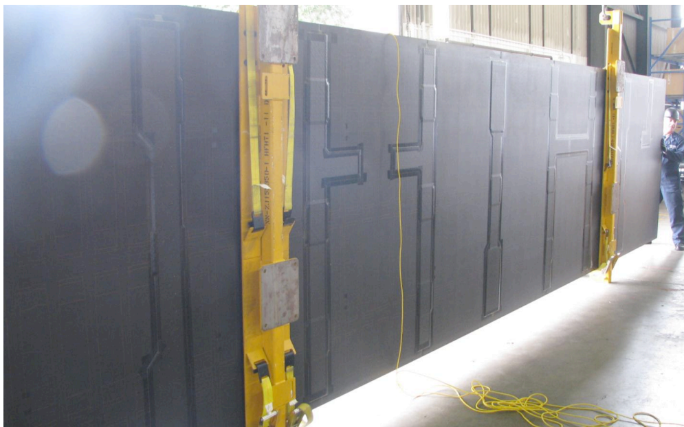
Figure 54. Completed Bonded Repair Patches on Crown Panel OML
