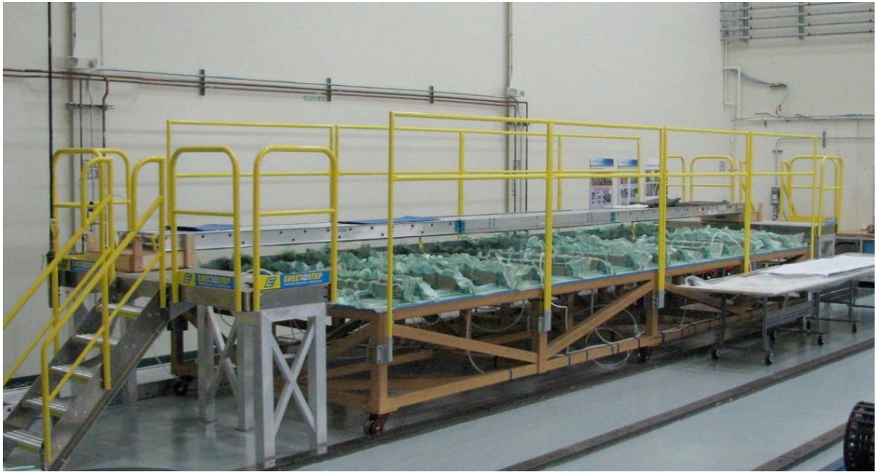
Figure 90. Upper Bulkhead Panel Preform Fully Bagged and Ready for Infusion
