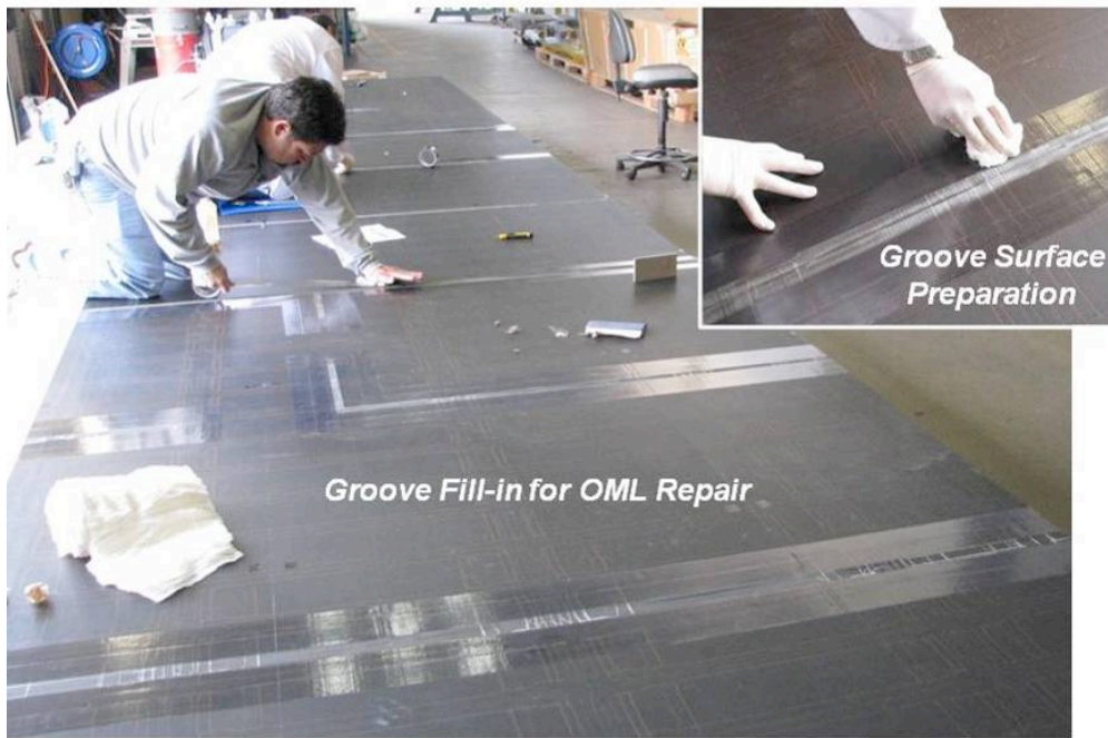
Figure 49. Crown Panel OML Surface Prepared for Repair
