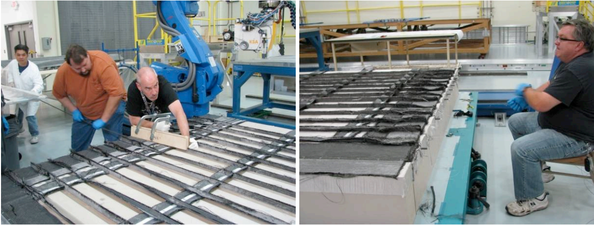
Figure 84. 30-ft Rods were Inserted into the Preform
