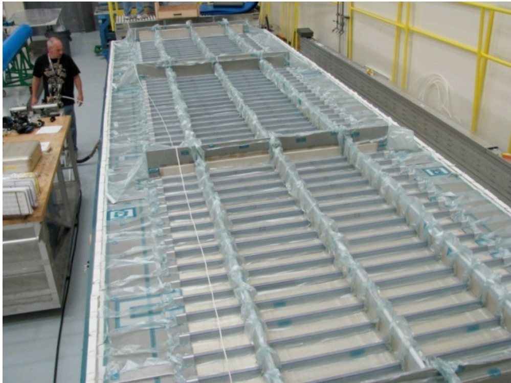
Figure 61. Primary Bag Installed and Leak Checked
