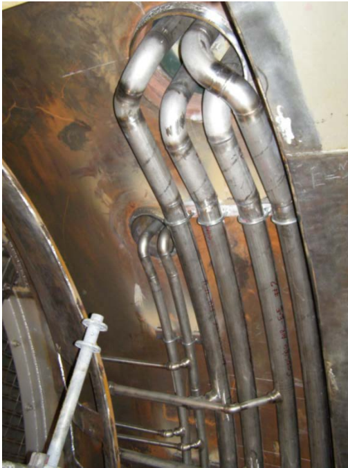
Figure 9. Plenum penetration.
