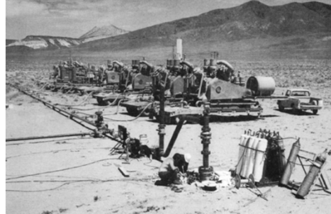
Field Measurements of Alluvium Permeability. Air Injector Setup at subscale hole. [9]
