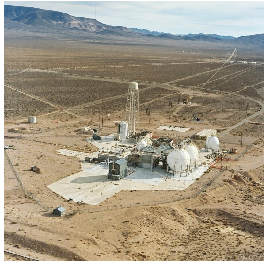
Test Cell "C"
