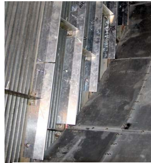
Figure 6. Cooling Coil Trailing Edge Fairings
