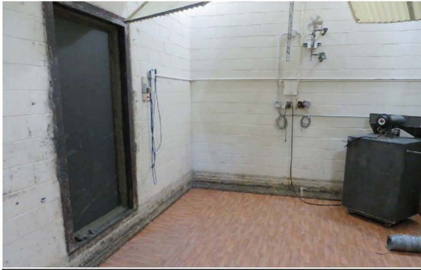
Figure 1 - The mounted FRF Panel as seen from the source room.
