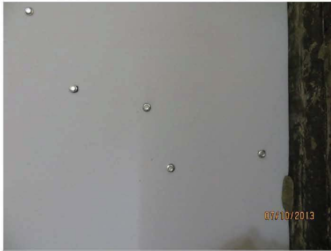
Figure 3 - Detail of penetrations filled with bolts.
