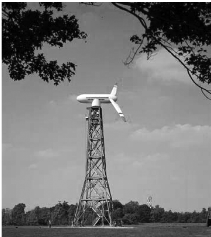
Figure 7.—Wind turbine at Plum Brook Station.
