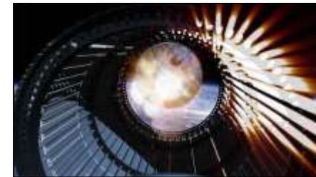
Internal stiffeners in spent fuel tank
