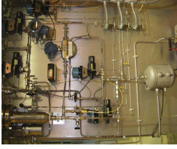
Green Propellant Flow Panel
