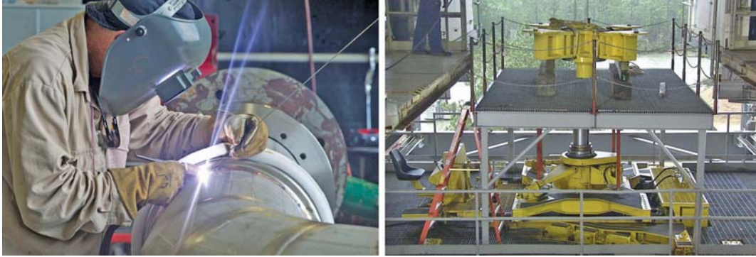
Fig. V: Renovating the SSC A-1 test stand (left) and RS-25 thrust frame adapter (right)
