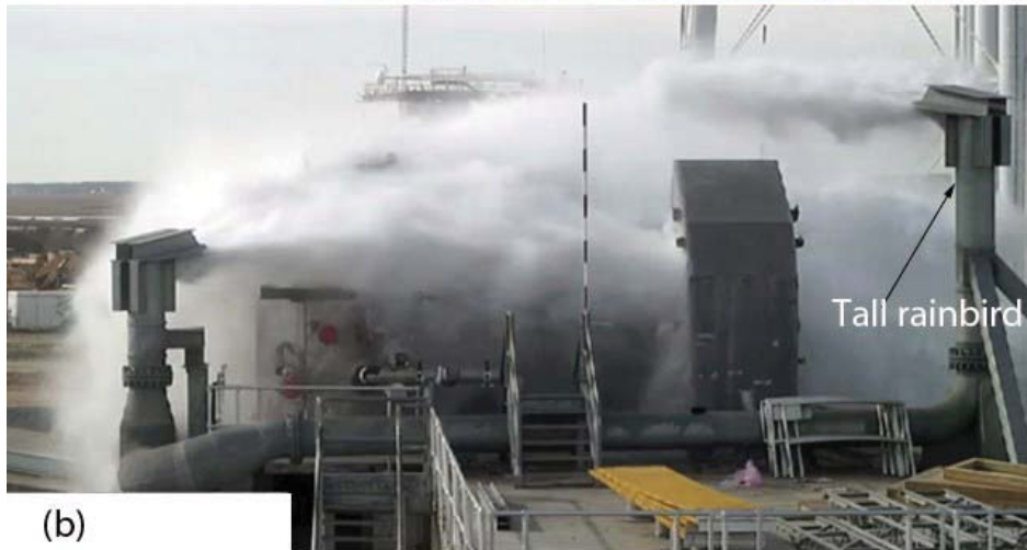
Fig. 2 Water injection systems used for acoustic attenuation in launch pad 0A. (a) Duct inlet water (view from the south-west side); (b) on-deck “rainbird” water (view from the east side).
