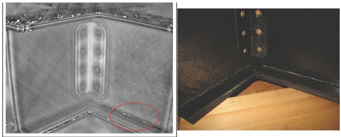
Figure A-25. Thermal inspection results for cruciform 2, rivet 1 bottom.
