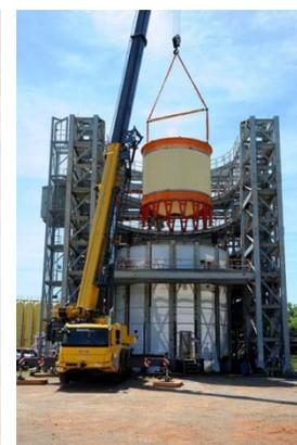
*5.5m tank arrives at MSFC for testing*
