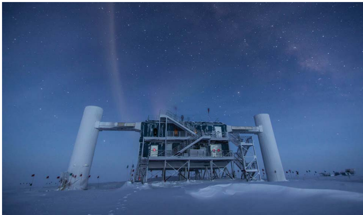
IceCube, located at the Amundsen-Scott South Pole Station in Antarctica, is the world's largest neutrino detector. The facility instruments a volume of roughly one cubic kilometer of clear Antarctic ice with 5,160 sensors at depths between 1,450 and 2,450 meters. The laboratory building shown here hosts the computers that collect the raw data. Credit: Felipe Pedreros. IceCube/NSF
