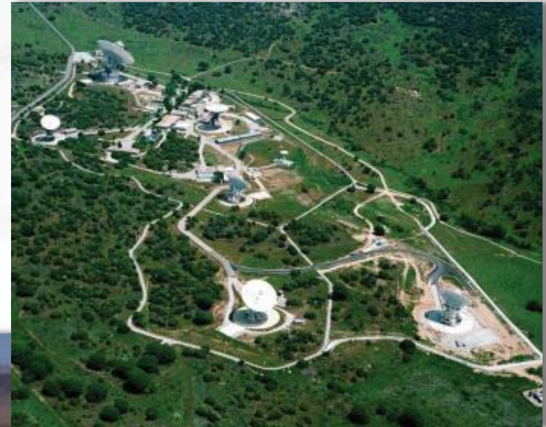
Madrid Deep Space Communications Complex
