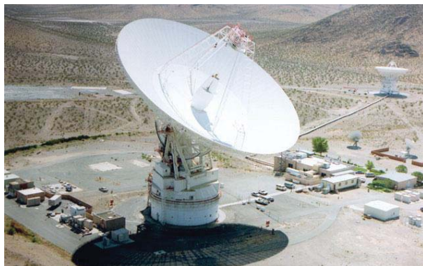
Fig. 1: 70-m dish (DSS-14) radar facility in Goldstone, California (Credit: NASA/JPL).
