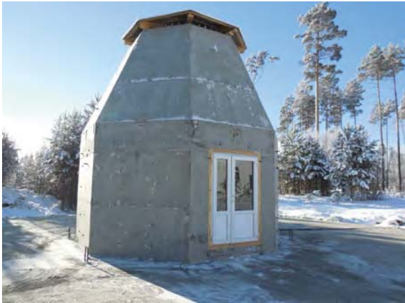
Fig. 5 Antenna tower for 13.2-m dish.
