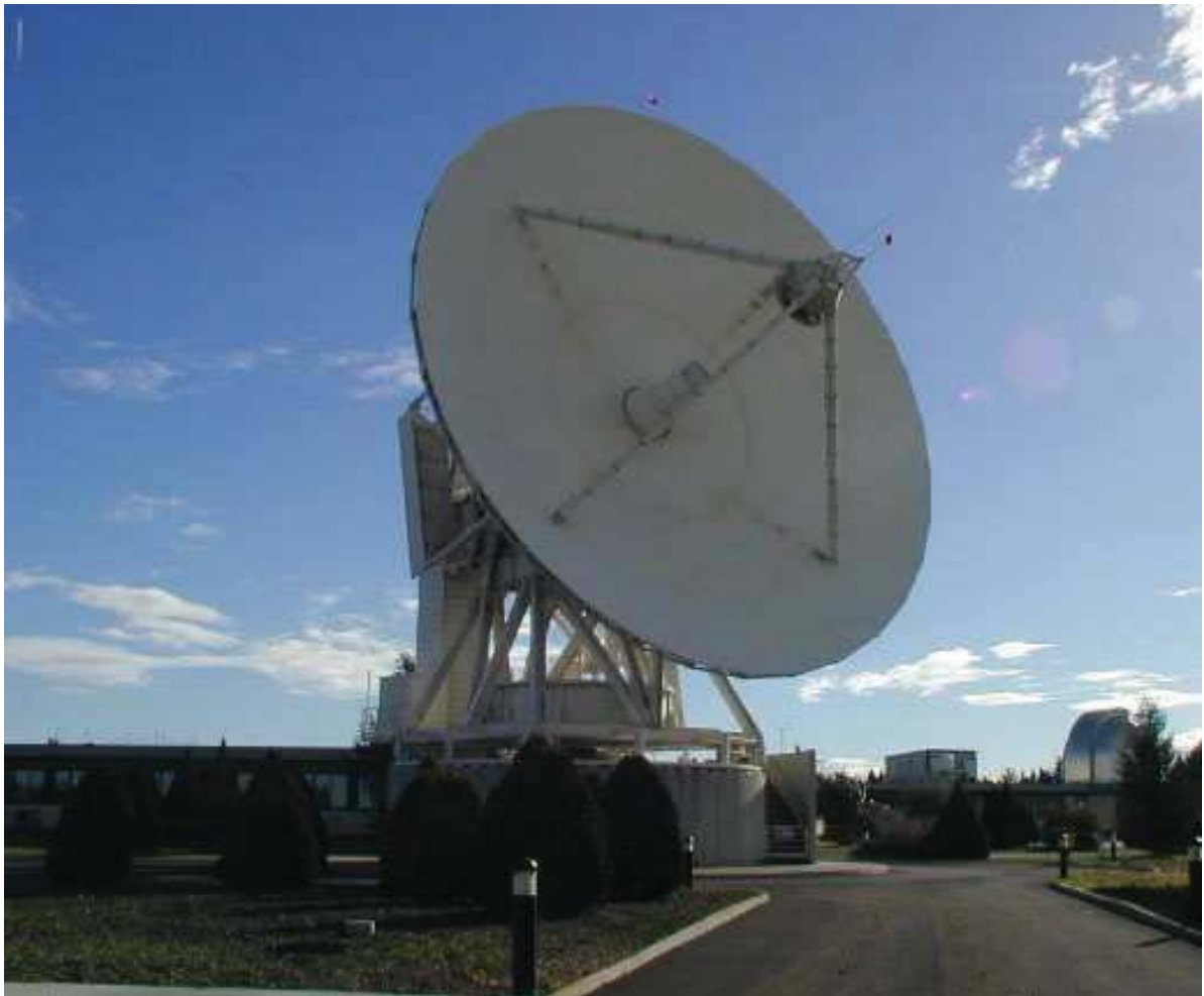
Fig. 1 VLBI antenna and MLRO dome.
