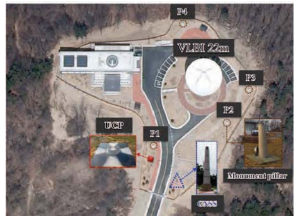
Fig. 1 Layout of the VLBI 22-m antenna, monument pillars 1 to 4, GNSS and UCP (Unified Control Point).
