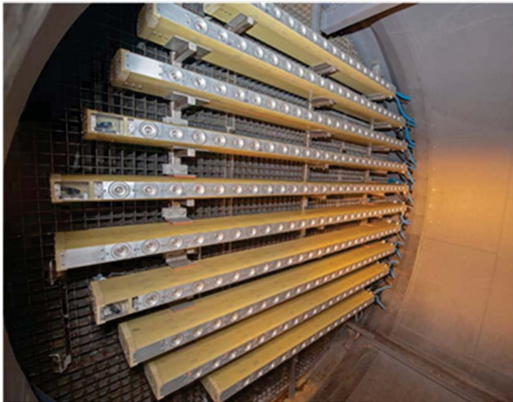
Figure 3. Water injection spray bars installed into the PSL cell three.
