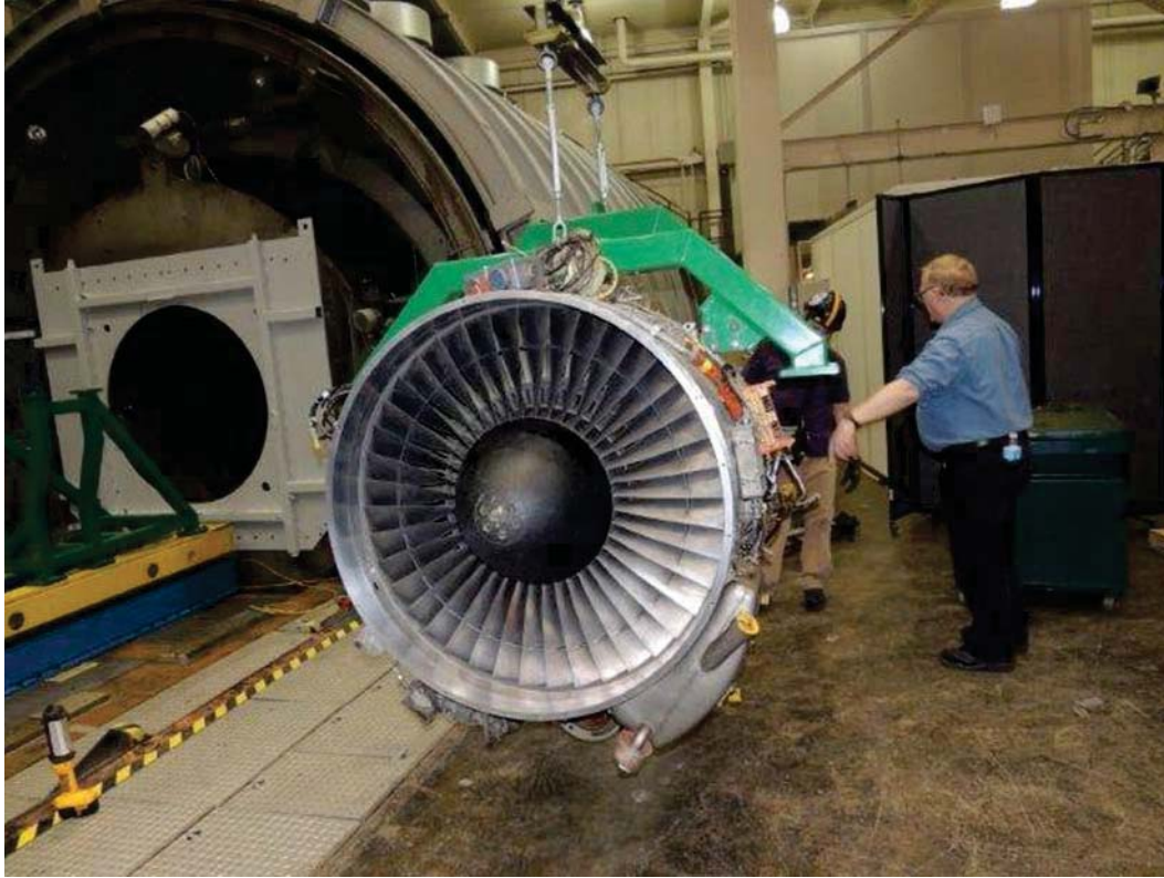
Figure 5. The ALF502-R5 (S/N LF01) engine being installed into PSL-3
