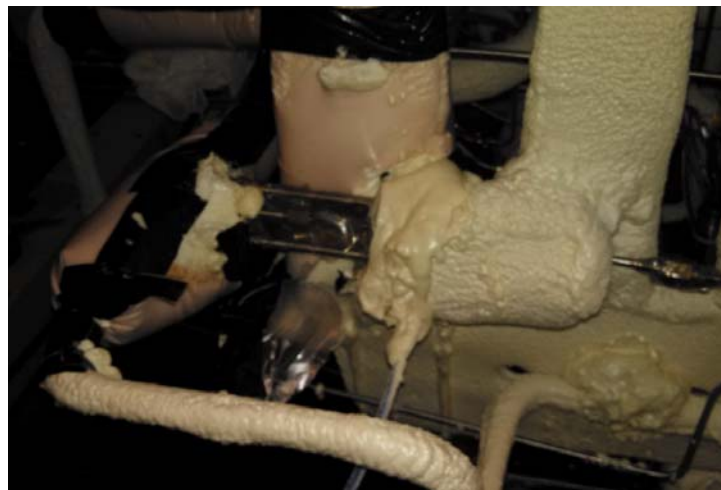
AFT Press Valve Closeout
