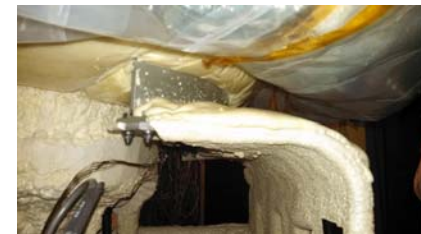
Mount Bracket Integrated to the Tank
