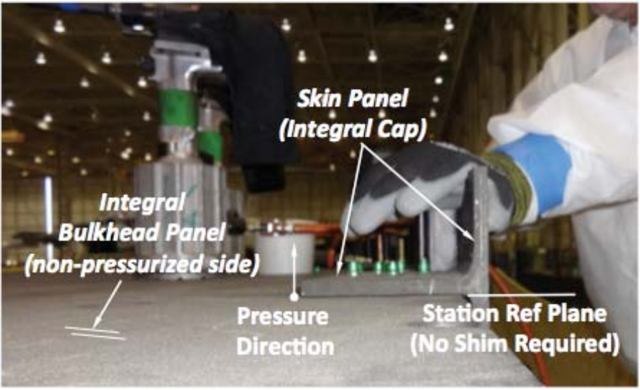
Figure 12. Molded integral cap station plane surface is used to locate panels.
