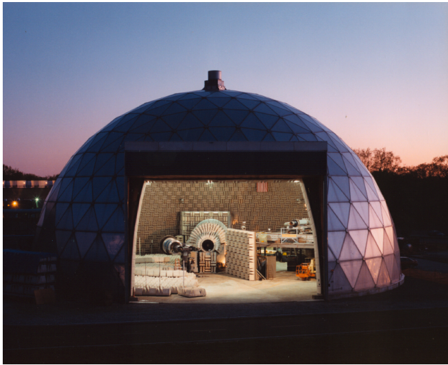
Figure 1. Aero-Acoustic Propulsion Laboratory
