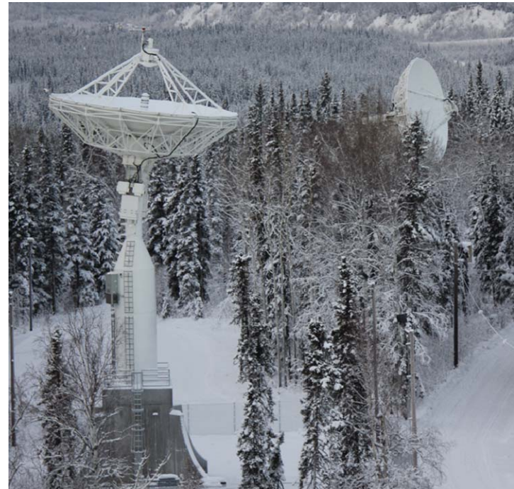
Near Earth Network Alaska Satellite Facility 11 Meter class antennas
