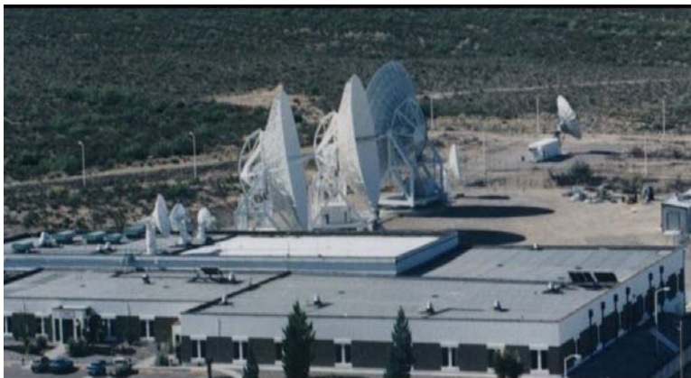
White Sands Ground Terminal (WSGT)
