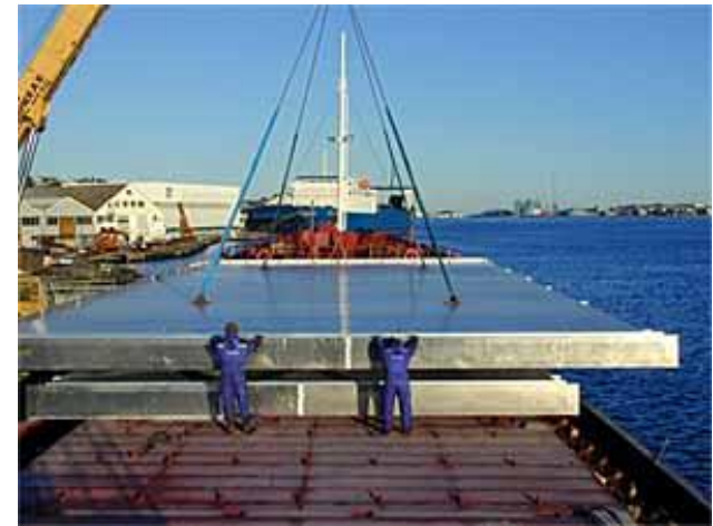
Prefabricated Deck Panels [7]
