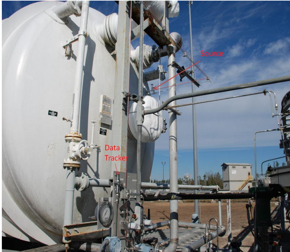
SSC Transducer Installation on LN2 Dewar
