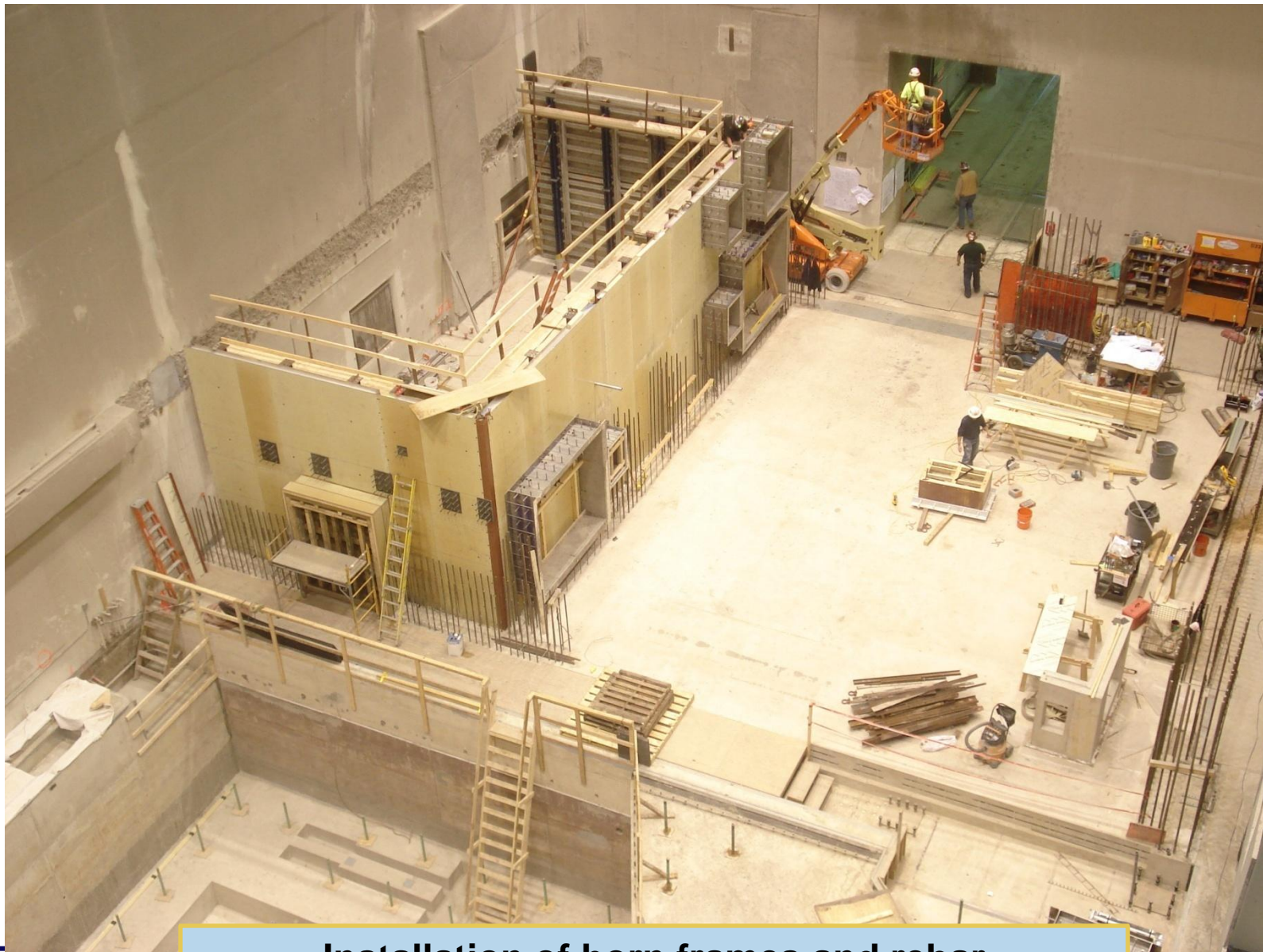
Installation of horn frames and rebar
