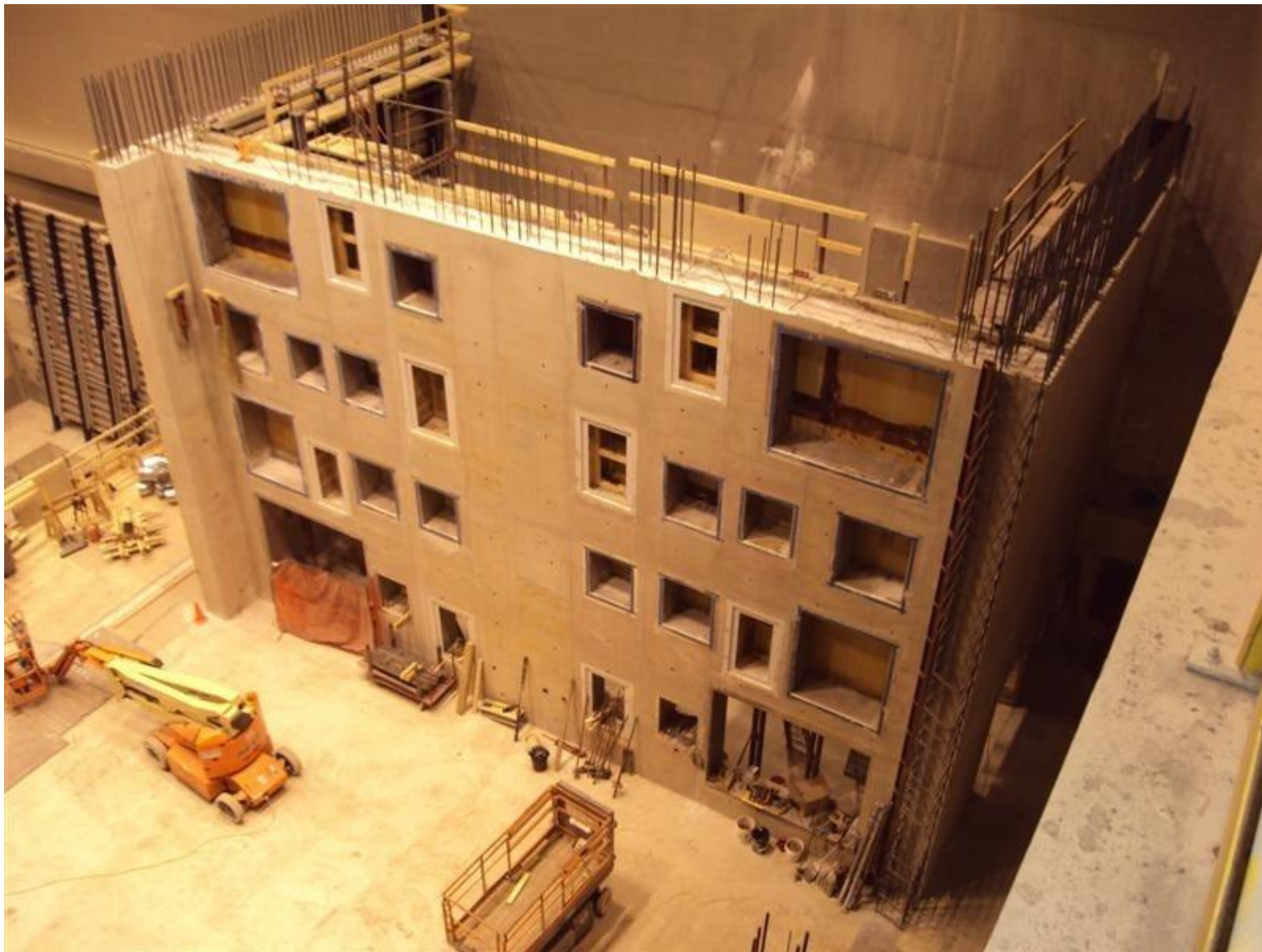
Concrete pour #2 completed with forms removed
