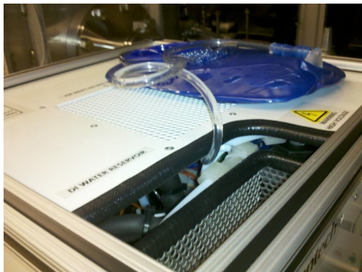
Figure 21.—Water reservoir for deionized water.
