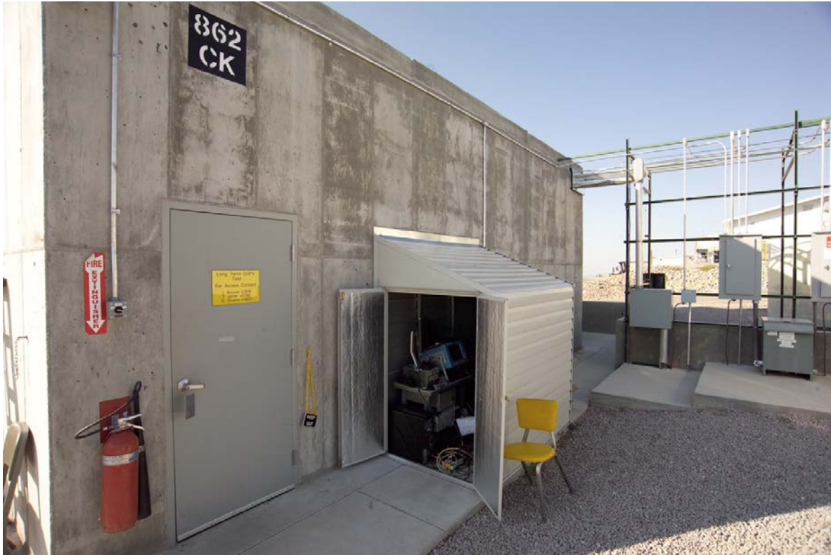
Figure 18 Electronics Isolated from a Potentially Catastrophic Event
