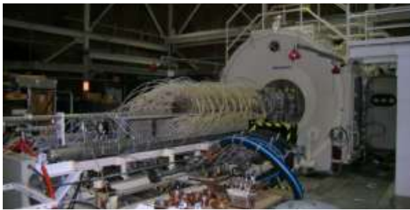
Figure 3: NASA JSC Arc Jet Test Facility
