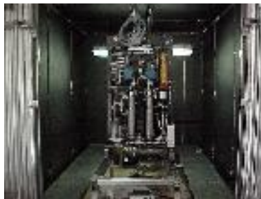
Sabatier/Water Electrolysis w/ CO 2 Absorption (LMA & JSC) [Tested under simulate Mars surface conditions]
