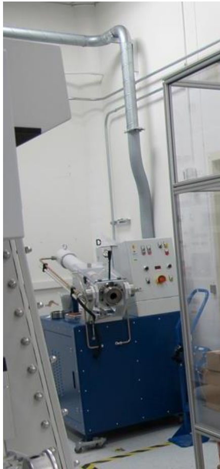
Graphite FE extruder with installed vent lines for DU capability
