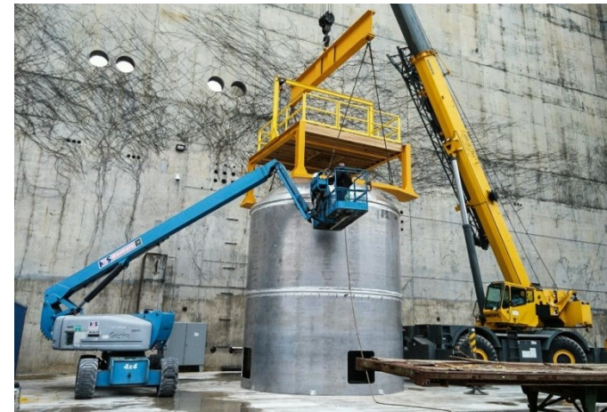
Placing the integrated test article on the test pad
