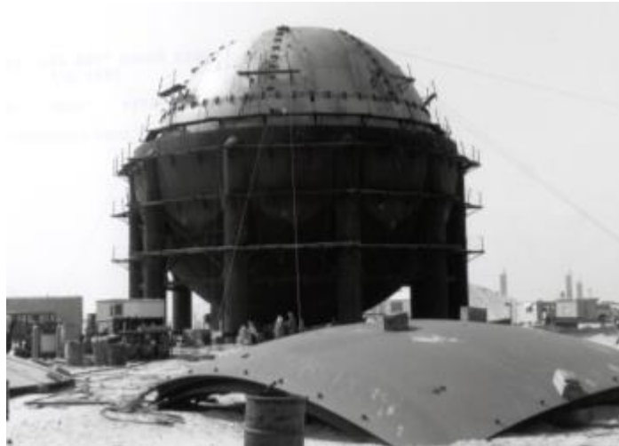
Figure 1. Construction of an 850,000 gallon LH 2 Sphere at LC-39
