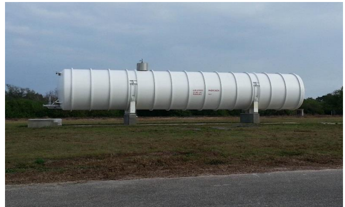
FIGURE 1: 33,000 GALLON LH 2 STORAGE TANK USED FOR GODU-LH 2
