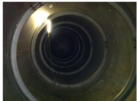
FIGURE 7: STIFFENING RINGS PRIOR TO STRINGER INSTALLATION & FINAL ADJUSTMENT
