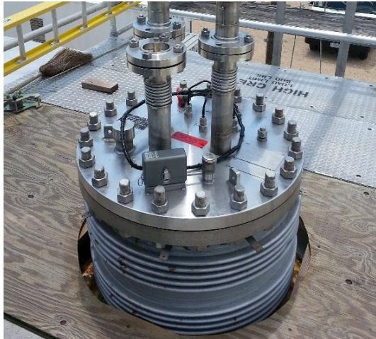
FIGURE 13: UPDATED MAN-WAY PLUG ASSEMBLY POST-MODIFICATION TESTING
