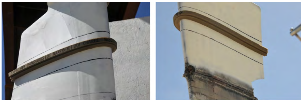
Figure 8.—Blade with shape charge around full circumference.
