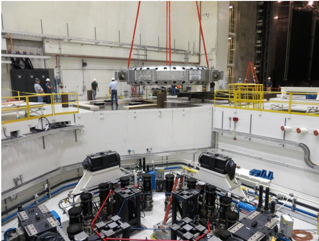
Fig 4 MVF Table (Above) Separated from MVF Pit (Below) Containing Actuators and Support Structure
