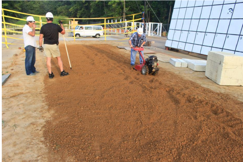
Figure 27 – Preparing the soil surface prior to Test 3
