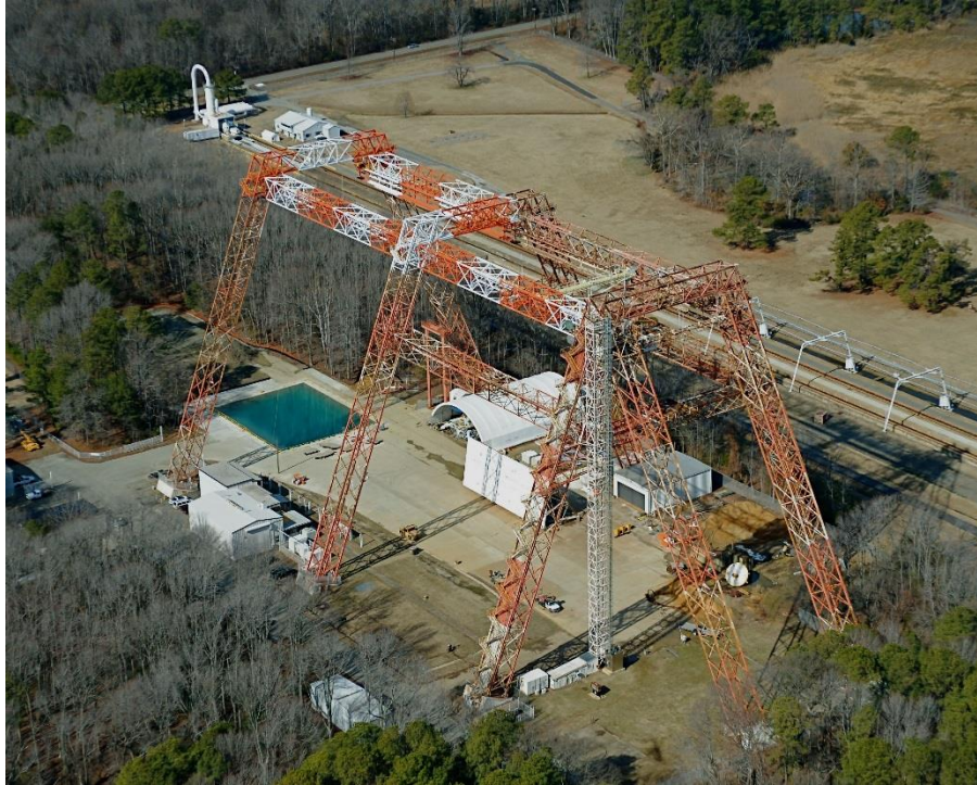
Figure 1 - Landing and Impact Research Facility (LandIR)
