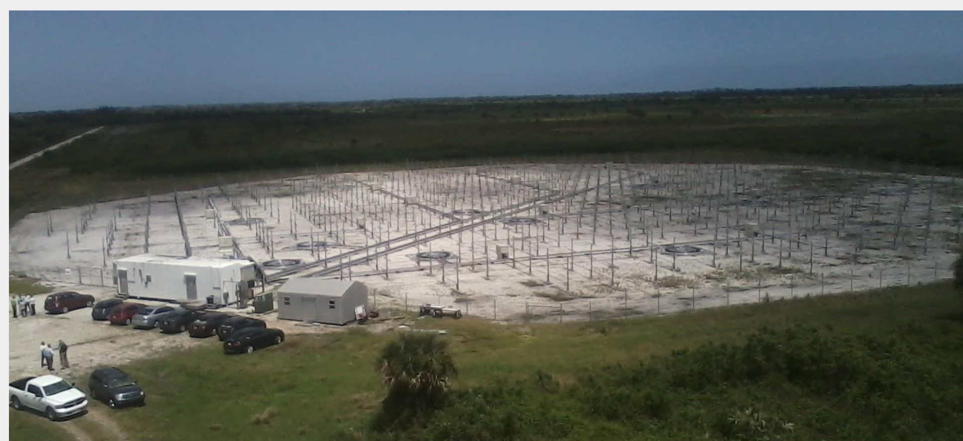
Figure 1: View of the new DRWP during installation.
