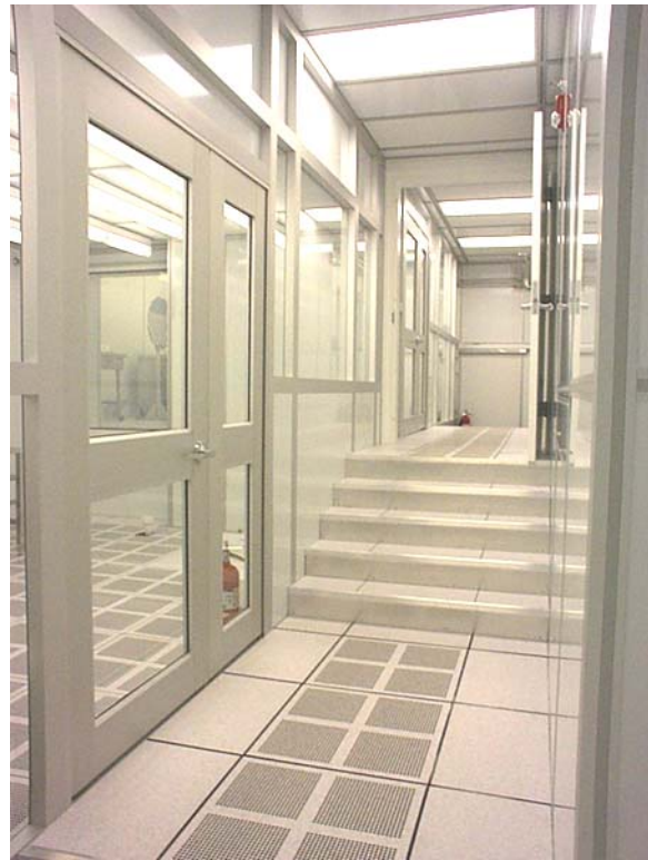
Fig. 5-5. Class 1000 Viewing Corridor provided quality observation opportunities without compromising the Class 10 cleanroom. Observers were required to don full cleanroom suits.
